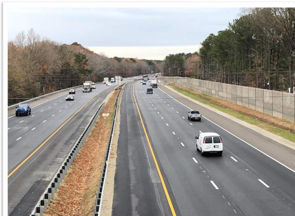
Project Site (Looking West from Denbigh)
