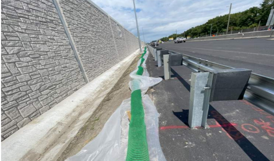
◀ Segment 4 Concrete Ditch and Guardrail
