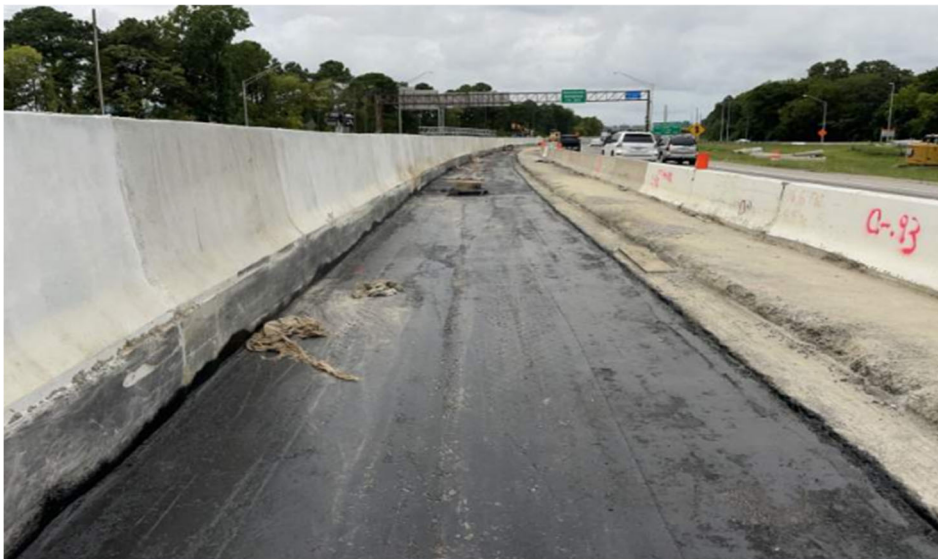
◀ Segment 1 CTA Placed and Tacked (Westbound Median)
