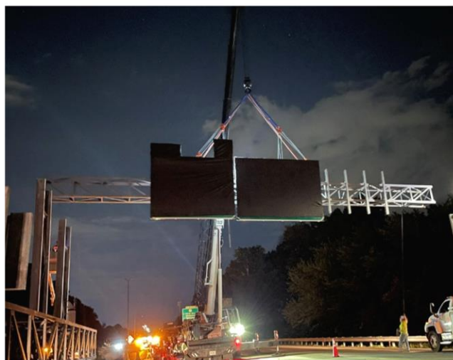
Overhead Sign Structure Installation
