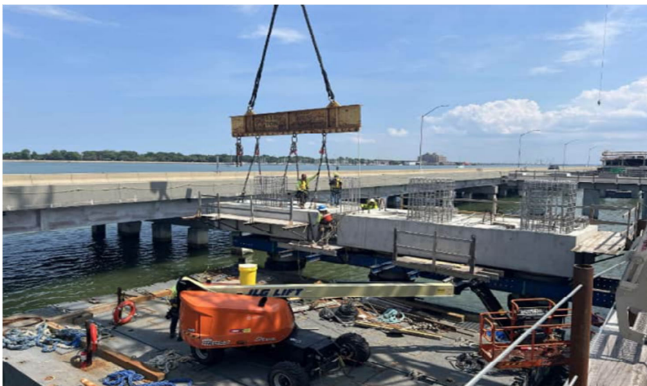
◀ North Trestle Westbound Installing Bent 7 Cap
